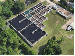
The City owns, operates, and maintains Castlebridge WWTP, with a permitted average daily flow (ADF) of 800,000 gpd or 0.8 MGD and a 2-hour peak flow of 1,885 gpm, with a peaking factor of 3.4.
