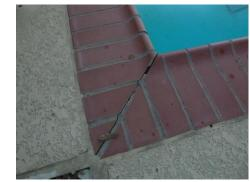
Figure 1.13, Coping stone cracking
