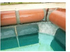
Figure 1.7, Coping stone loose and cracking Figure 1.8, Area of corner wall repair
