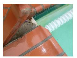
Figure 1.11, Loose/unsecured coping stone
