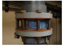
Figure 1.39, Piping bolt corrosion
