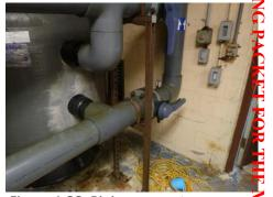
Figure 1.28, Piping support corrosion | area of filter leak
