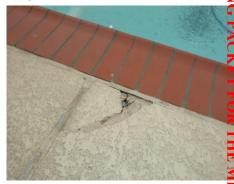
Figure 1.16, Pool deck delamination
