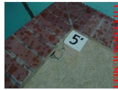
Figure 1.14, Pool deck delamination
