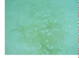
Figure 1.4, Plaster surface etching/delamination
