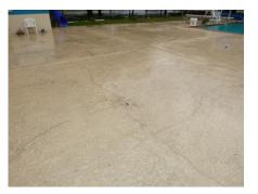
Figure 1.19, Pool deck cracking
