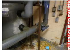
Figure 1.34, Piping support corrosion | area of filter leak
