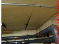
Figure 1.42 Mechanical room ceiling damage
