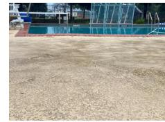
Figure 1.12, Uneven/shifting concrete deck and pool
