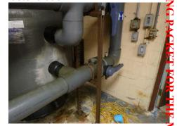
Figure 1.40, Piping support corrosion | area of filter leak
