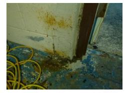
Figure 1.29, Wall/door deterioration
