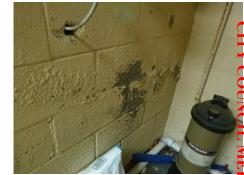
Figure 1.38, Mechanical room wall deterioration
