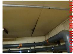
Figure 1.36, Mechanical room ceiling damage
