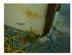
Figure 1.41, Wall/door deterioration
