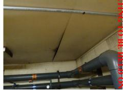
Figure 1.30, Mechanical room ceiling damage
