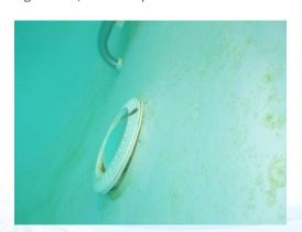
Figure 1.5, Underwater light not in place
