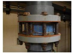
Figure 1.33, Piping bolt corrosion
