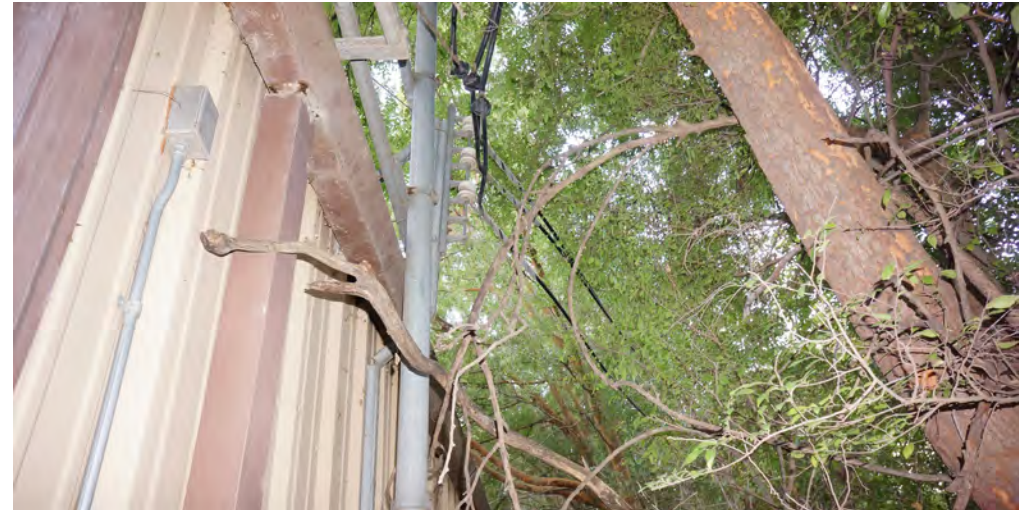
Tree vegetation has grown so much that it interferes with the Golf Course Cart Barn's power source.
