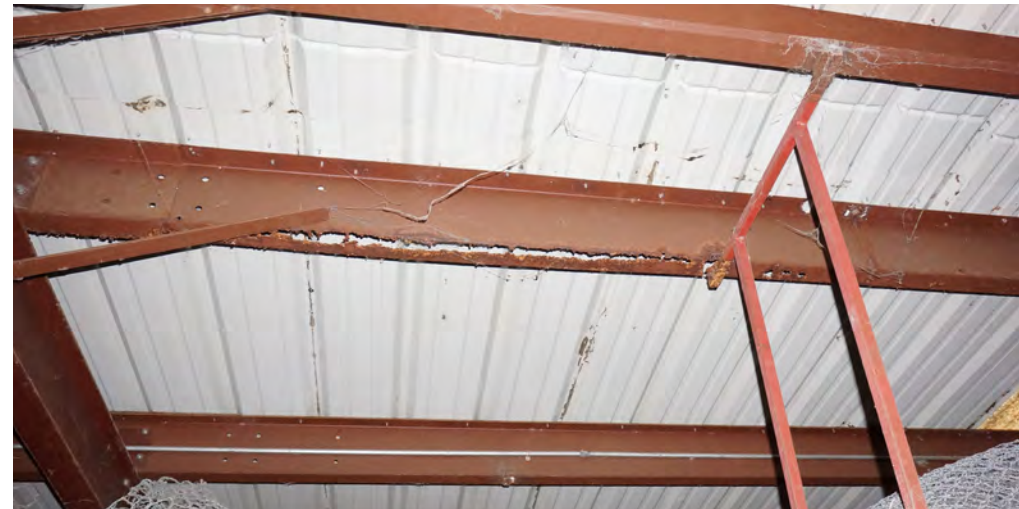
Structural members show signs of major corrosion.
