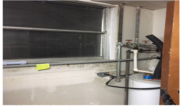
Mold at Gyp board
