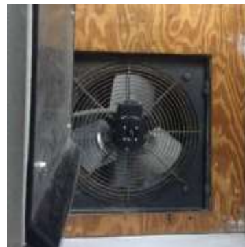
Assumed Outside Air Fan Not Operational
