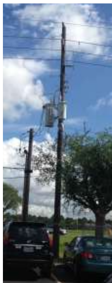
Pole Mount Transformer
