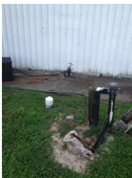
4" PVC Sanitary Sewer Cleanout
