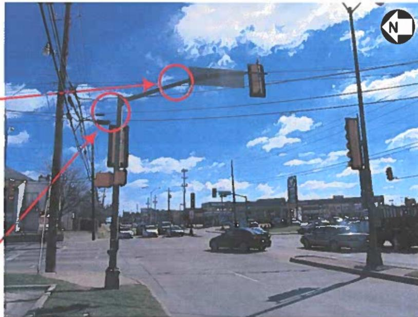
Install equipment enclosure here with cover facing north.
