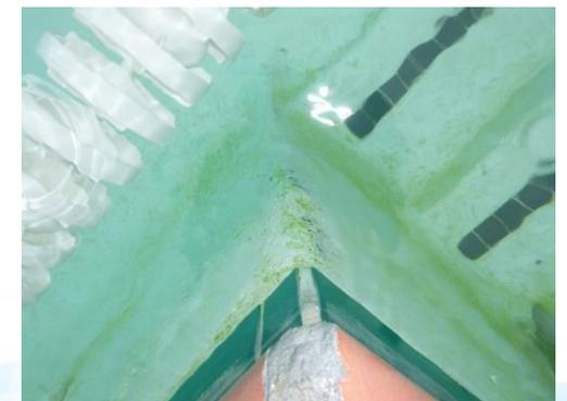
Figure 1.6, Cracking, delamination on corner
