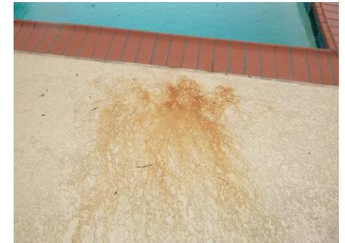
Figure 1.18, Pool deck corrosion
