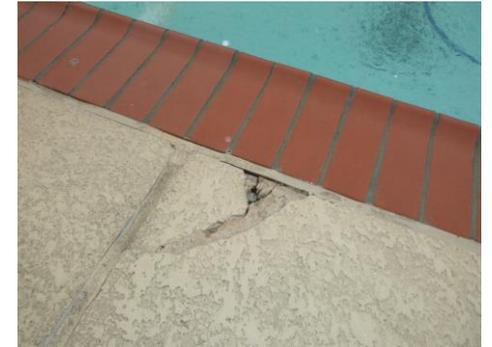
Figure 1.16, Pool deck delamination
