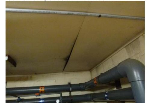
Figure 1.42 Mechanical room ceiling damage
