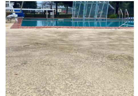
Figure 1.12, Uneven/shifting concrete deck and pool
