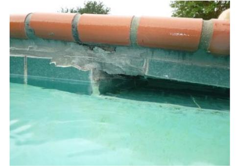
Figure 1.10, Cracked, shifting skimmer basket
