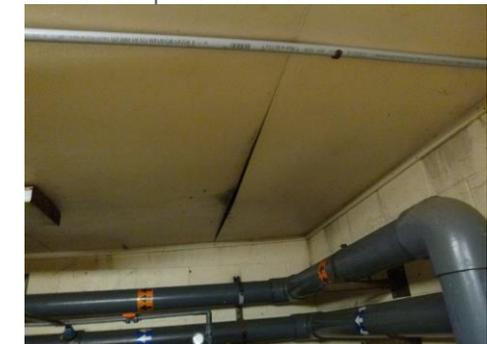
Figure 1.30, Mechanical room ceiling damage
