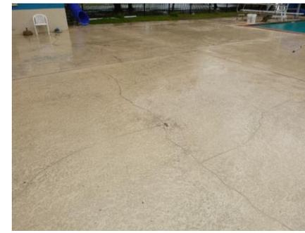
Figure 1.19, Pool deck cracking
