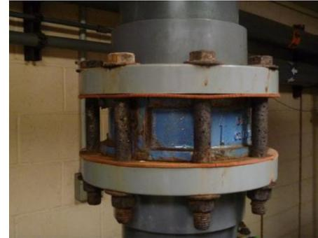
Figure 1.39, Piping bolt corrosion
