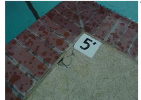
Figure 1.14, Pool deck delamination
