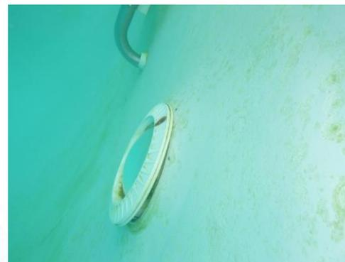
Figure 1.5, Underwater light not in place
