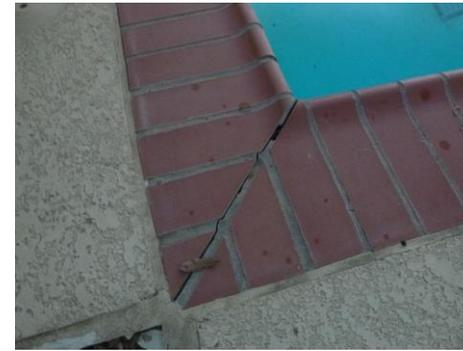
Figure 1.13, Coping stone cracking
