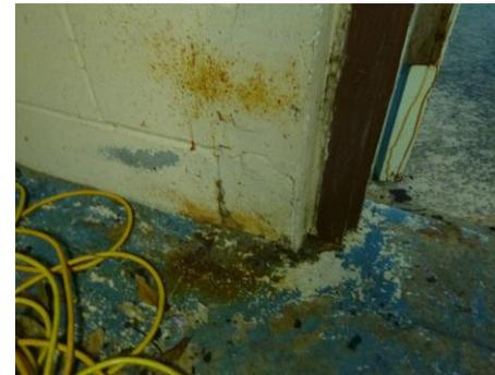
Figure 1.41, Wall/door deterioration
