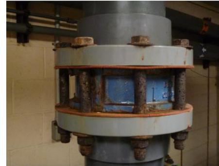
Figure 1.33, Piping bolt corrosion
