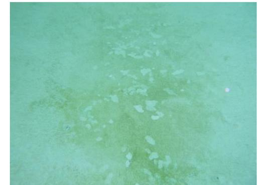
Figure 1.4, Plaster surface etching/delamination
