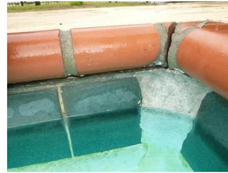
Figure 1.7, Coping stone loose and cracking
