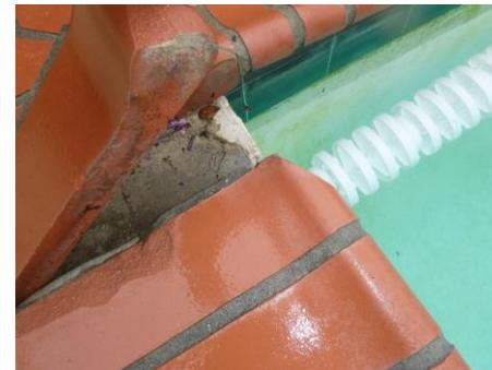
Figure 1.11, Loose/unsecured coping stone
