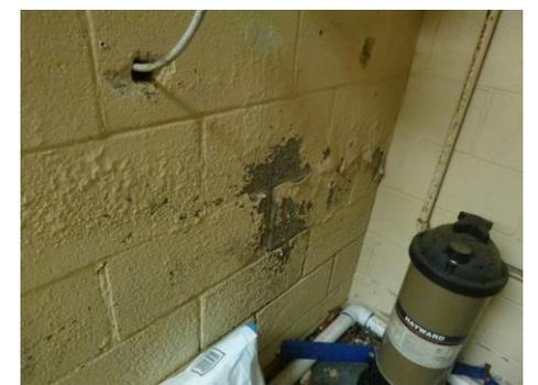
Figure 1.38, Mechanical room wall deterioration
