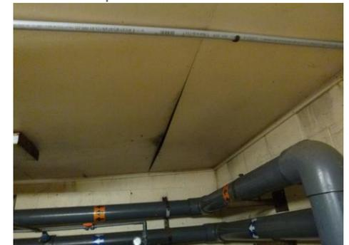
Figure 1.36, Mechanical room ceiling damage
